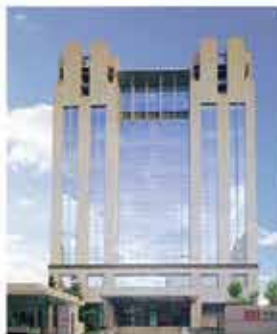
MEAN WELL GUANGZHOU TIANHE R&D CENTER
